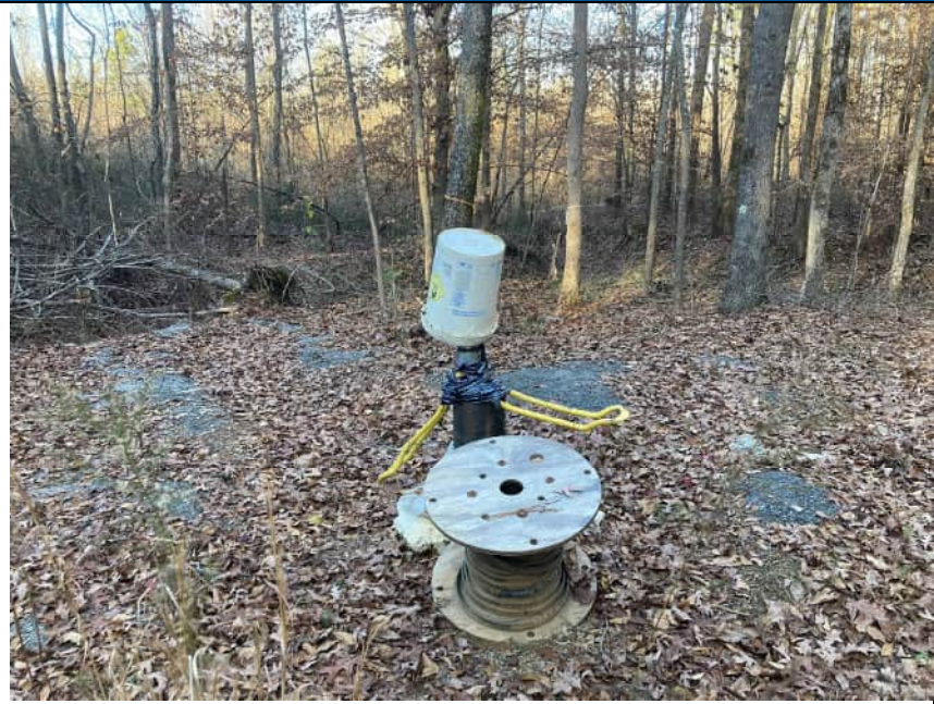
Photo 1: Well #4 area. Bucket is positioned on top of outer casing.
